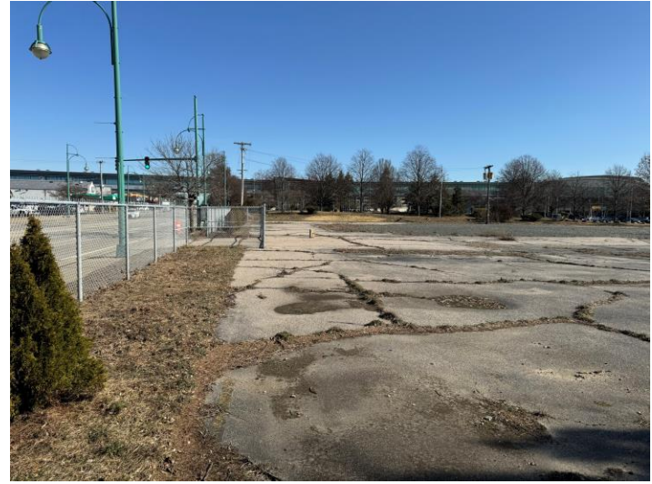
PP3 looking north
