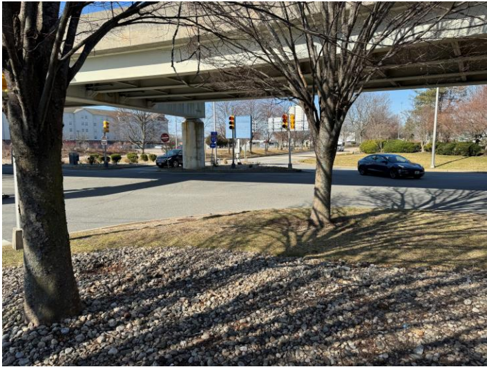
PP7 looking west
