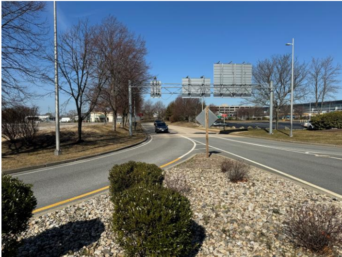
PP8 looking west
