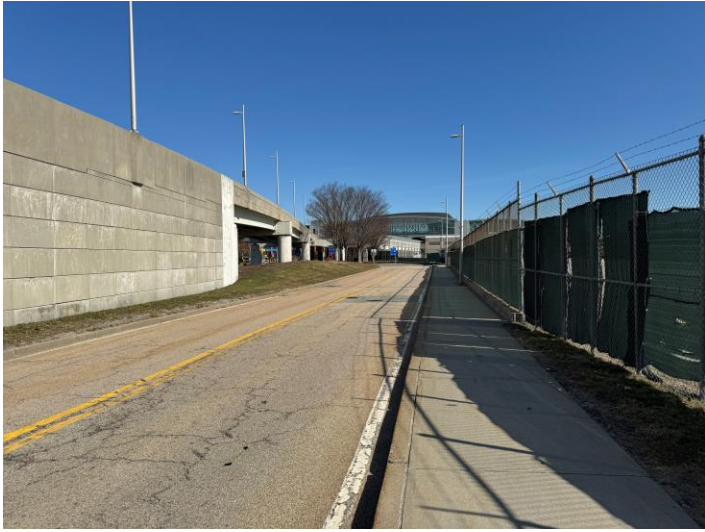
PP6 looking north
