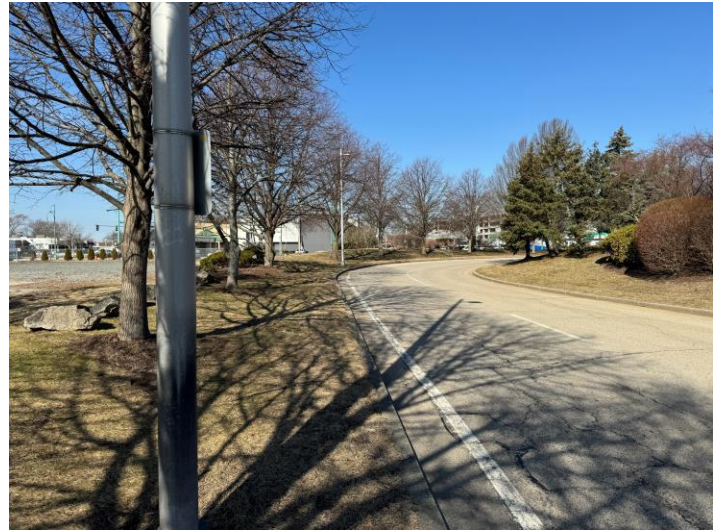
PP5 looking west
