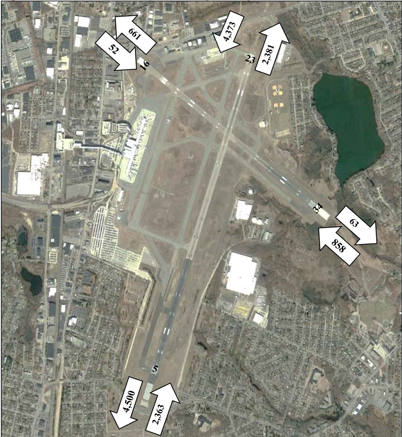
Figure 2: Aerial View of Total Operations, by Runway End, 4th Quarter, 2022
