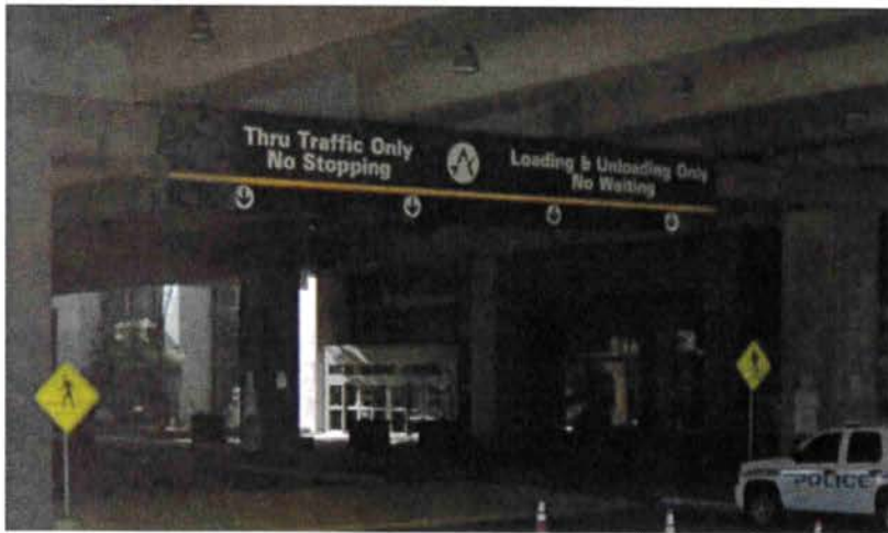
Figure 6.27: Overhead Lane Assignment Signage, Austin Bergstrom Int'l Airport
